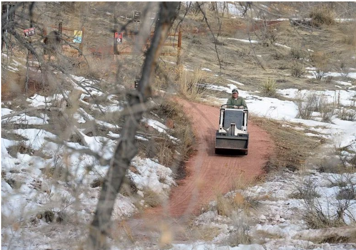
David Slater, Larimer County trails employee, uses a walk-behind bobcat to fix a dip on the trail Friday, Dec. 19, 2019, at the Devil’s Backbone open space in Loveland. (Jenny Sparks/Loveland Reporter-Herald)
