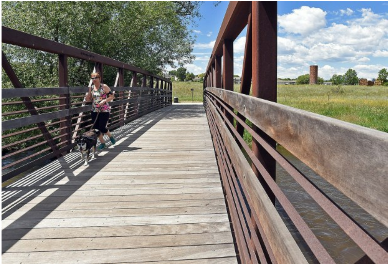
LOVELAND, CO – JUNE 13, 2019: Liane Weinberger and her dog, Kailie, run across a bridge on the Poudre River Trail on Thursday, June 13, 2019, at the River Bluffs Open Space in Windsor. (Photo by Jenny Sparks/Loveland Reporter-Herald)
